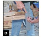
Once positioned so that the joist is in line with the final chalk line, fasten through both the plate and bracket perforations in an offset triangle fashion to ensure solid anchorage of the stamped bearing bracket into position (See G).
