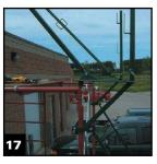
19 Install all additional diagonal braces and safety guard rails as outlined on the engineered specifications (fig. 16 & 17).
