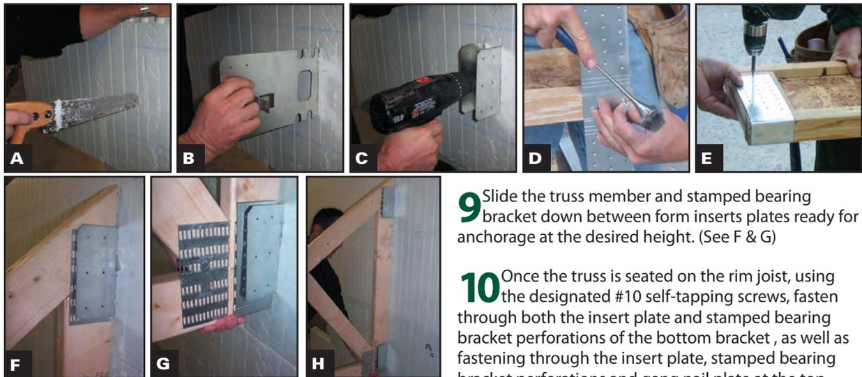
**9** Slide the truss member and stamped bearing bracket down between form inserts plates ready for anchorage at the desired height. (See F & G)
