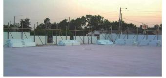
Special care should be taken to have form units accessible where needed while maintaining a 7' (2.13 m) clear distance around the perimeter of the walls to allow room for the alignment system installation discussed later in this chapter. Also a clean, accessible work site will prove to be beneficial both in terms of production and safety.
