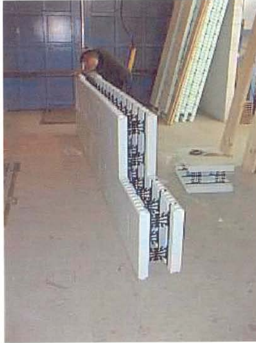
Photograph No. 1: Assembling of insulated concrete form wall modules
