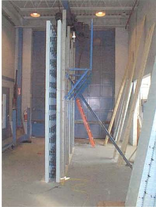
Photograph No. 3: Wall assembly with bracing attached.
