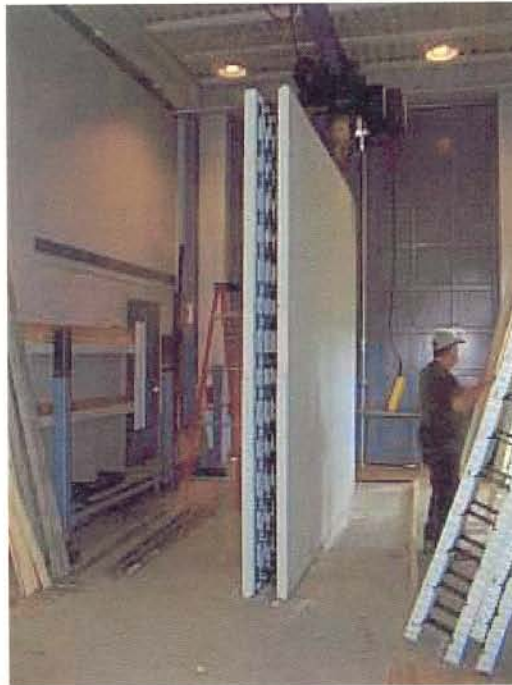
Photograph No. 2: Wall assembly before bracing and end caps installed.
