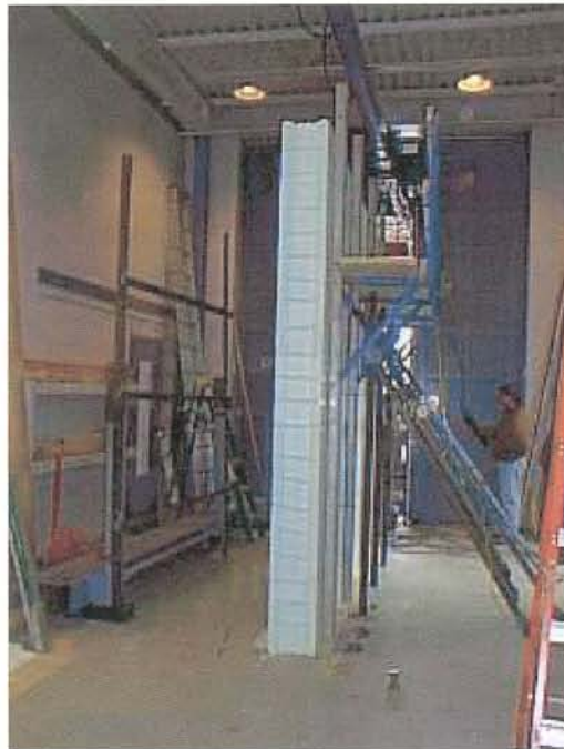
Photograph No. 4: Wall assembly before concrete pour.
