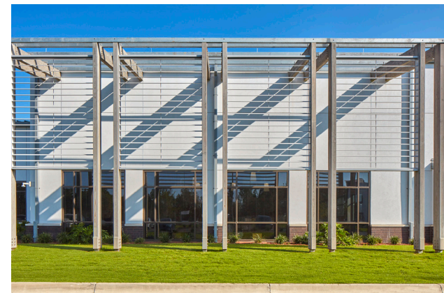
Dune Lakes Elementary School Santa Rosa Beach, Florida
